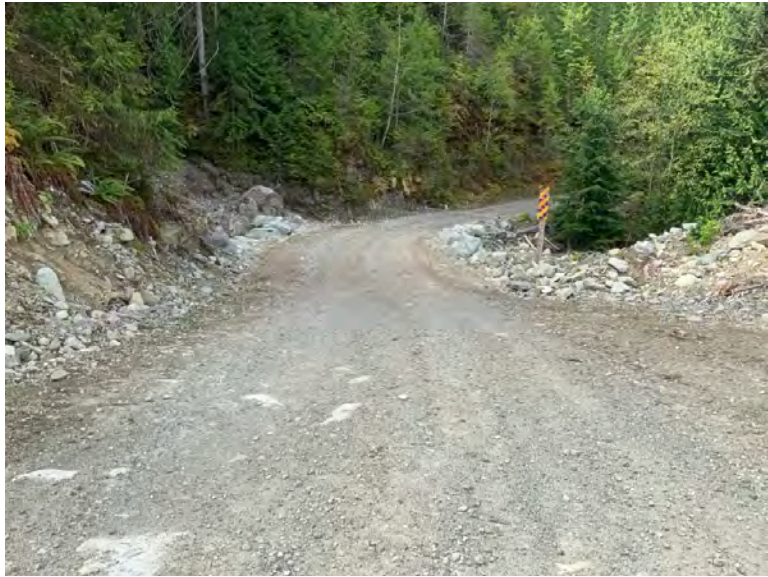
Approach from Right Bank when facing downstream
